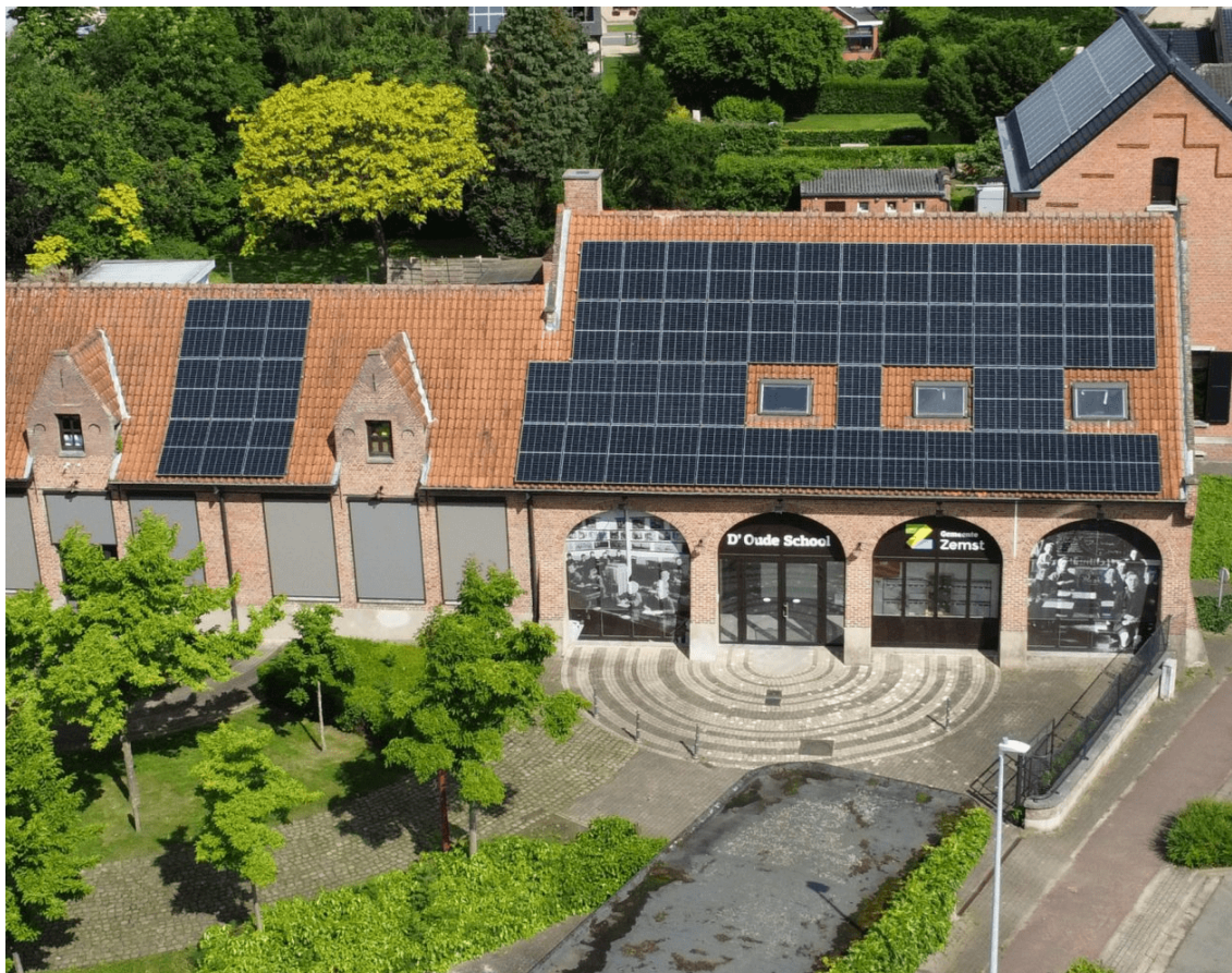
Solar PV installation of Klimaan on 'd Oude School, one of the Zemst community buildings
